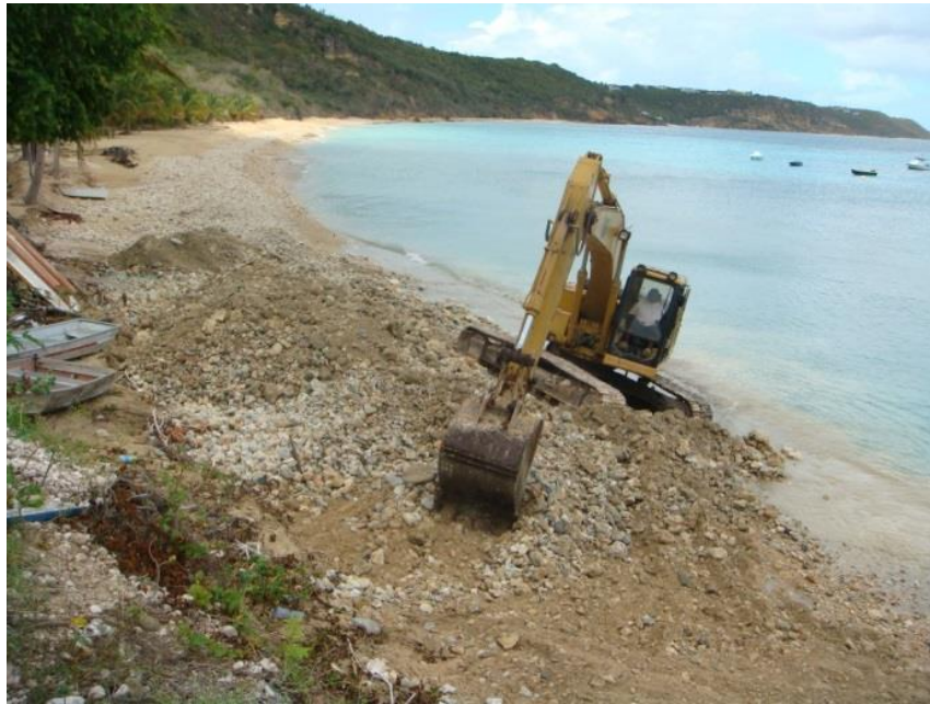
Plate 17 (left) Removal of stones at Crocus Bay uncovered by strong ground swells in early 2008. This material would have formed an important foundation for the beach here and a great defence against such sea conditions. Material was sold as aggregate. Photograph courtesy of DFMR archives.
