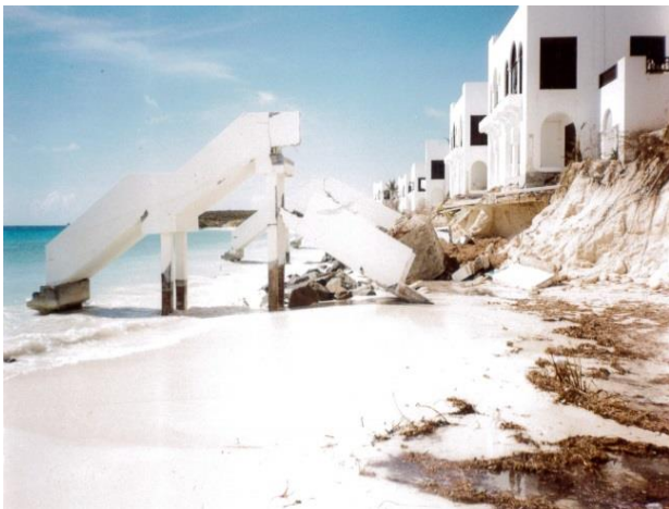
Plate 6 (left) Severe beach erosion at Maundays Bay following Hurricane Lenny in 1999. Much of the beach was washed away and villas undermined, leaving their access stairs as floating ‘islands’ in the wash zone. Photograph courtesy of Dr. G. Cambers.
