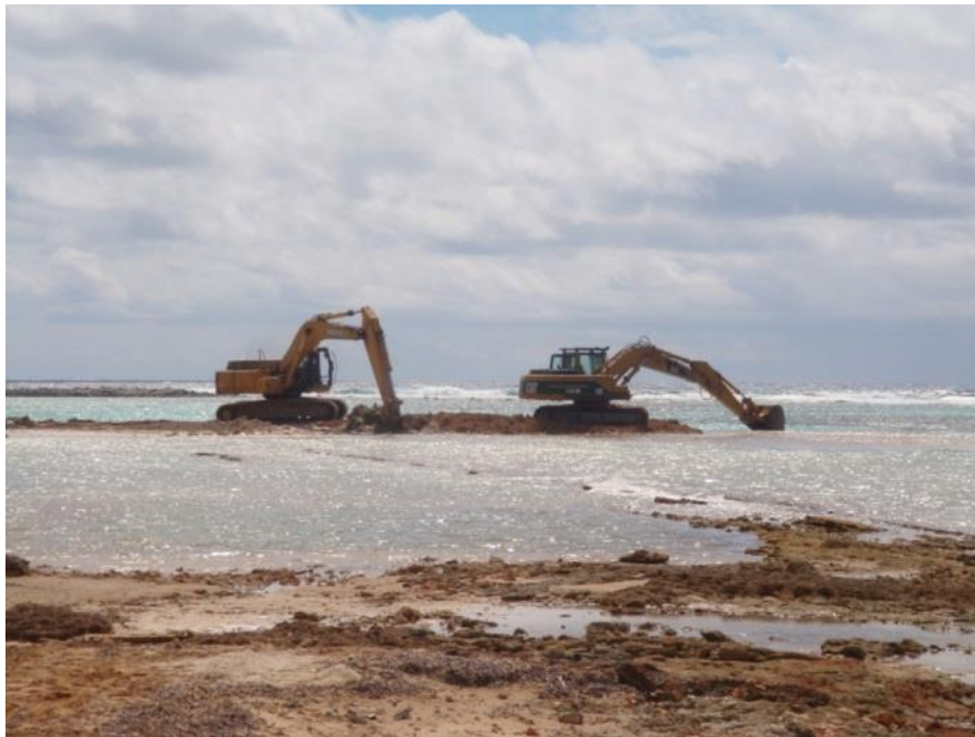
Plate 20 (right) Digging sand from within Forest Bay in April 2008 as an attempt to create a beach to convince investors for the potential of a new coastal resort development. Photograph courtesy of DFMR archives.
