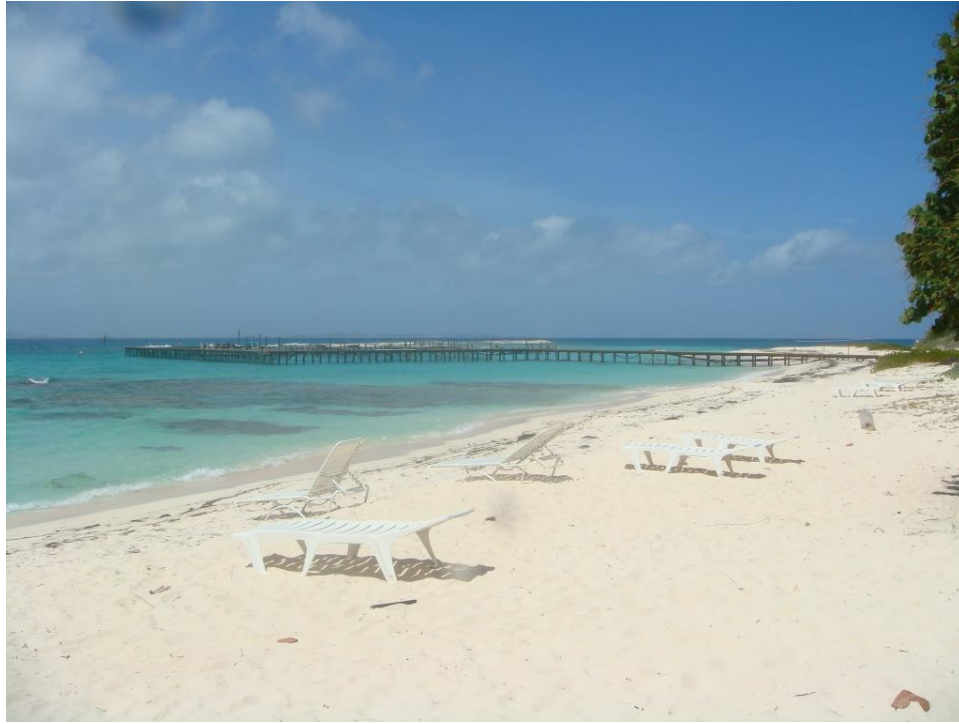
Plate 8 Dolphinarium under construction at Sandy Point in June 2008. The sand spit just beyond the construction is much reduced from that seen on older maps. Since the photograph was taken the spit has begun to extend seawards again. Photograph courtesy of S. Wynne.
